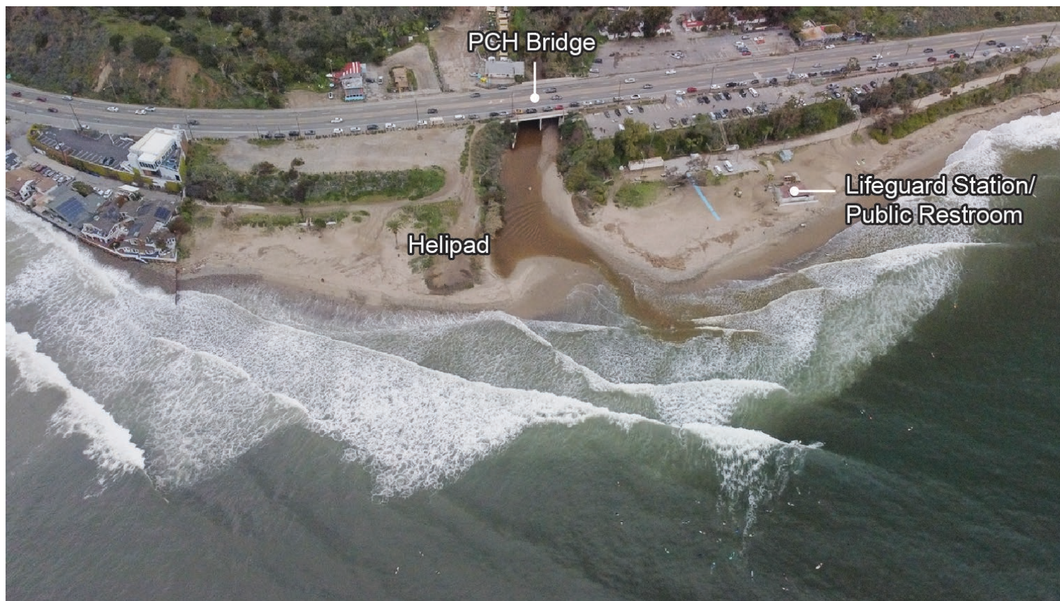
Topanga Lagoon Restoration Project
